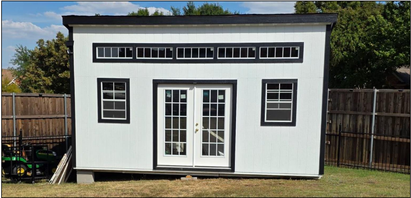
FIGURE 1: IMAGE OF THE UNPERMITTED ACCESSORY STRUCTURE
